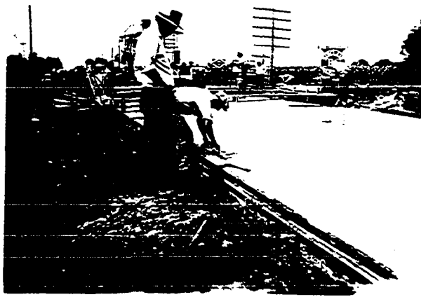
Smoothing the curb
