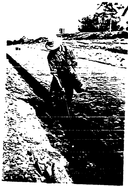
Protect the pavement edge with asphalt oil
